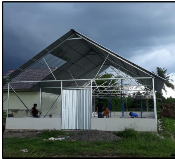
Figure 7: Stages of BSF Installation Construction
