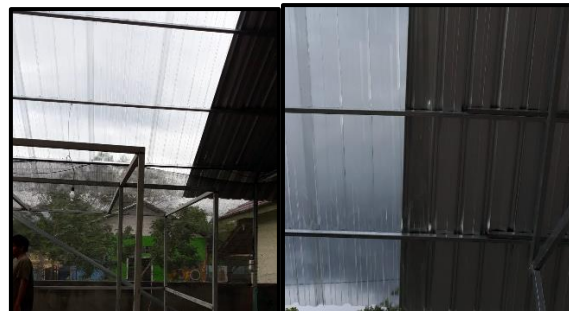
Figure 11: Installation of Flyhouse Transparent Roof
