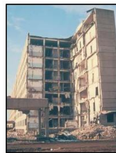
Figure 5: spitak Armenia earthquake (1988)
