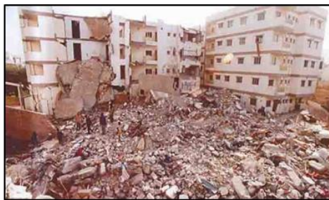
Figure 4: bhuj earthquake, India (2001)
