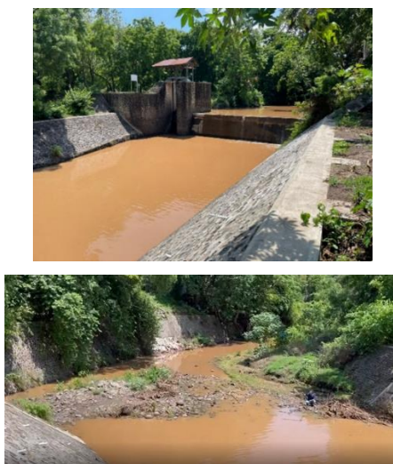
Fig 1: River conditions at the Kalokoran Dam
