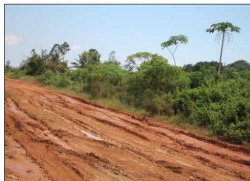
Road Condition of Paloh to districts Paloh
