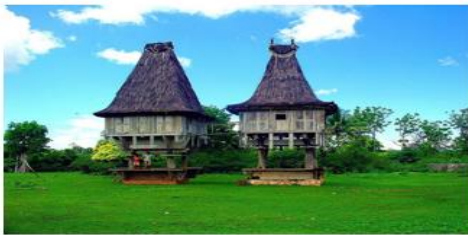
Figure 2: Typical Timor Leste Traditional House
