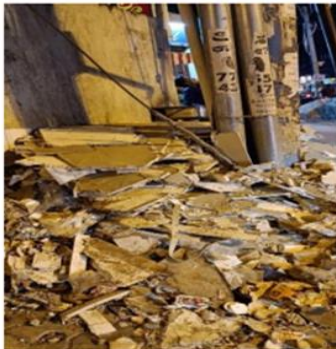
Fig 1: Waste POP gypsum Board dumped
