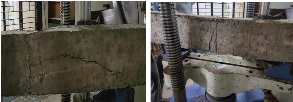
Fig. 4: Failure and cracking pattern of beams.
