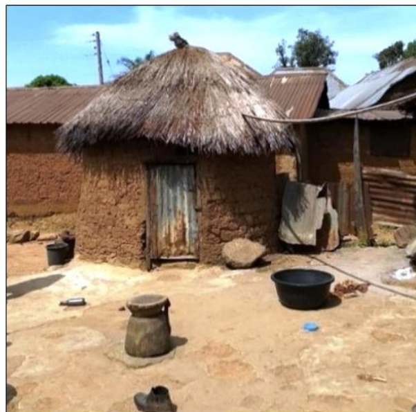
Figure 8: Pre-colonial Gbagyi courtyard in Karshi, Karshi Area Council
