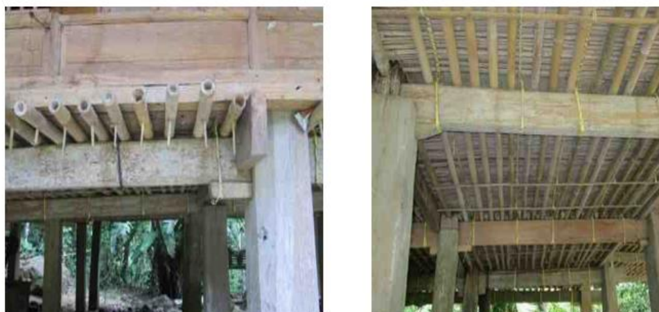
Fig 17: Dowel Connection System
