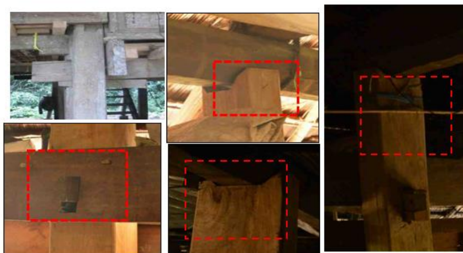
Fig 16: Connection Tie System Source: Field Survey, May 2022.
