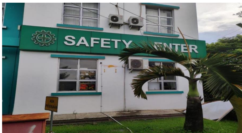
Figure 6: Safety Center Office of PT. Indonesia Power PLTU Barru OMU
