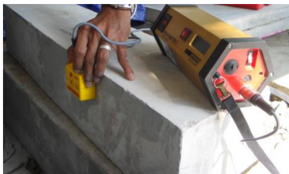
Figure 4: Mapping of reinforcement with profometer
